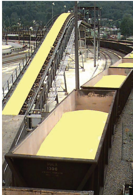
Sulphur handling at PCT
