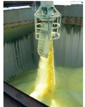
The 40-meter high shiploader allows 5,000 tons of sulphur per hour to be poured from the conveyor belt straight into a ship's hold.
